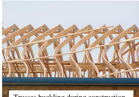
Trusses buckling during construction
